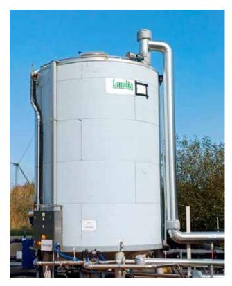
At the end of the process, in order to meet the legal requirements of a feedstock that contains animal bi-products, there are now two (25 m³) Landia pasteurisers, which heat the final effluent to the required temperature of 70 °C.
