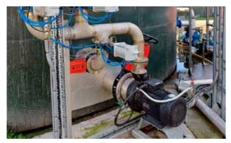
The new mixing system in question is a simple, but highly effective one. Externally-mounted, a Chopper Pump (invented by Landia in 1950) with venturi nozzles. No working at height. No working in the gas zone. And no costly downtime for servicing.
