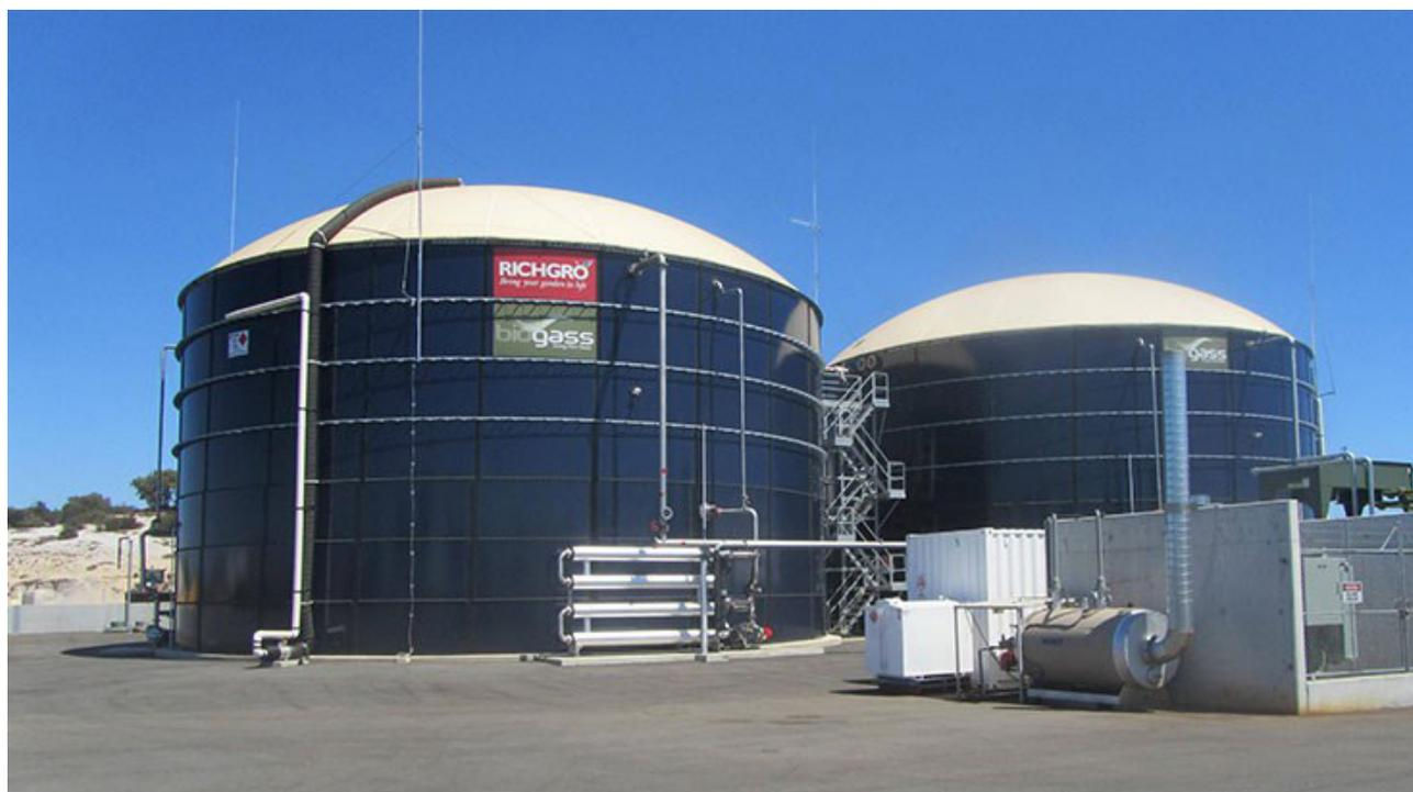
gasholders on the top, supplied and constructed by Biodome Asia, a Kirk Group subsidiary located in Selangor, Malaysia. In addition, Biodome Asia also supplied the 12,360 cubic feet open-topped blending tank, a 12,360 cubic feet feeding tank with steel roof and a 17,658 cubic feet digestate storage tank, also with steel roof.
