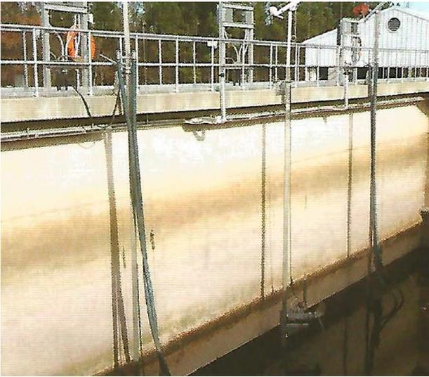
Landia mixers and jet aerators were installed to mix and aerate the thickened sludge (1% dry solids), to ensure a uniformed sludge solids concentration and to minimise anaerobic conditions.
