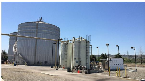
**The system is designed to help boost gas production at the Chino facility's two anaerobic digesters.**
