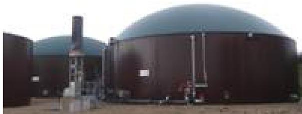
**Externally mounted GasMix systems, designed and manufactured by Landia, have helped Eco Sustainable Solutions increase the amount of biogas it produces by twelve and a half per cent.**
