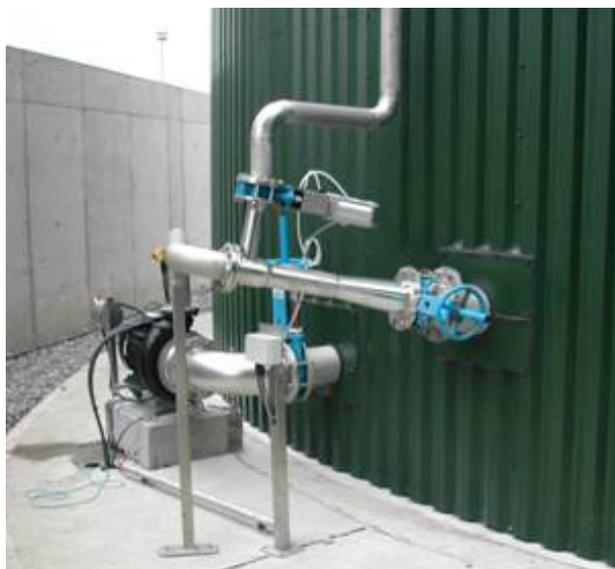
*Landia's externally mounted GasMix AD digester mixing at Tullamore WWTW*
