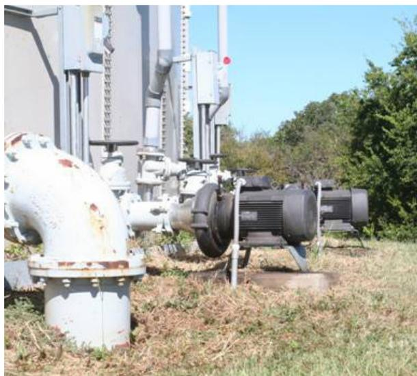
*Externally mounted chopper pump aeration system at Gun Barrel City*
