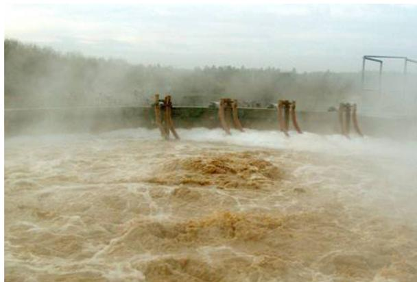
*This equipment provides simultaneous aerating and mixing.*
