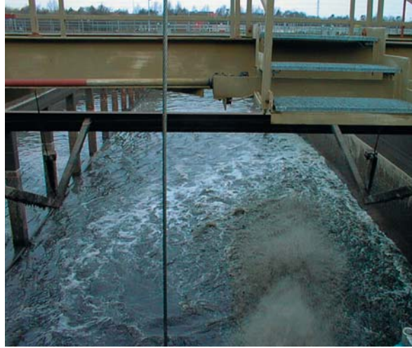
Storm water tank cleaning
