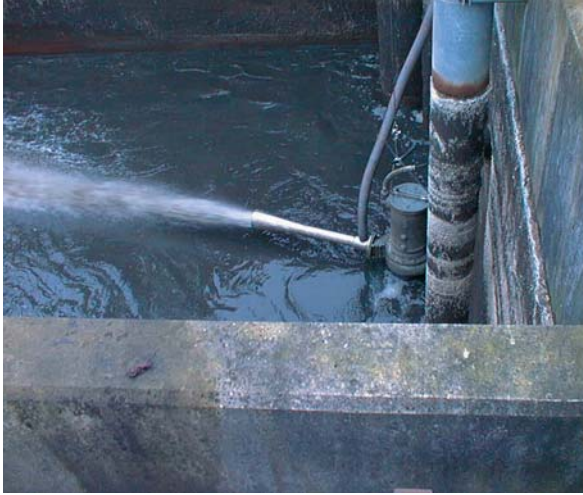
Storm water tank cleaning
